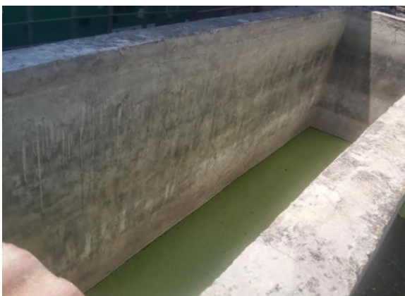
Step 4: Secondary settling (Secondary sedimentation tank)
