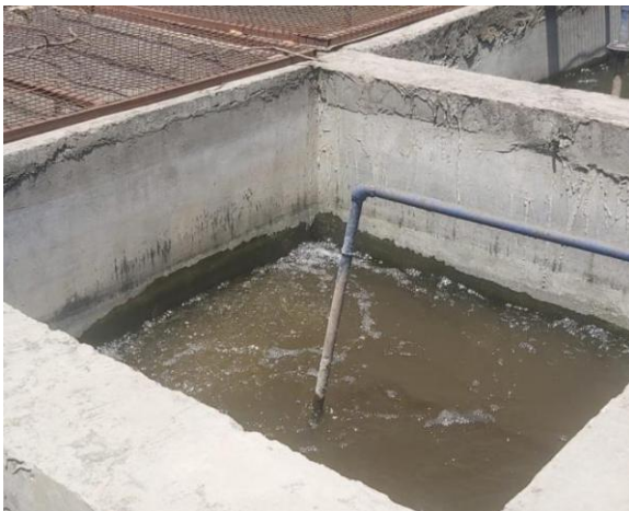
Step 3: Secondary treatment (Aeration / Activated Sludge)
