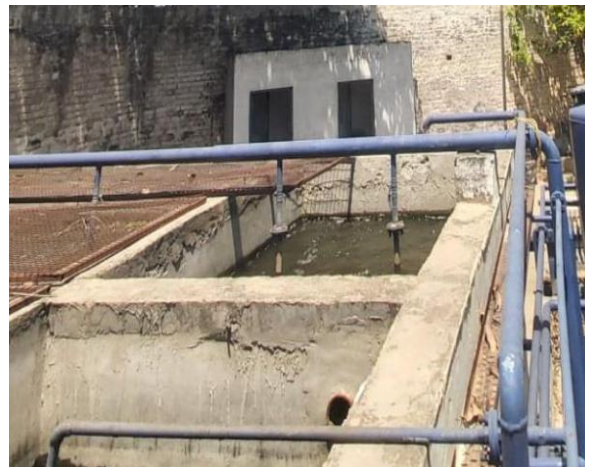
Step 2: Primary treatment (Primary sedimentation tank)
